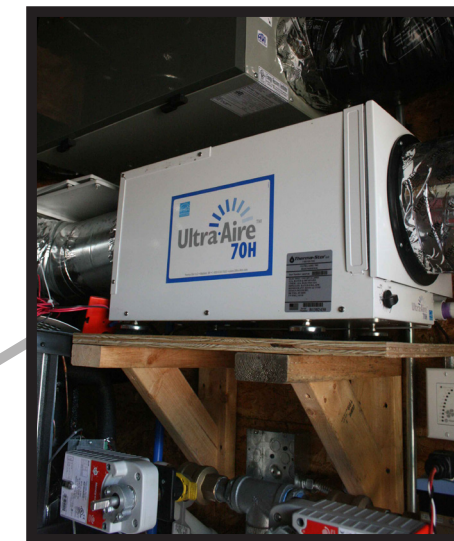
Building envelope integrated with passive and active systems and designed to Passivhaus standard
