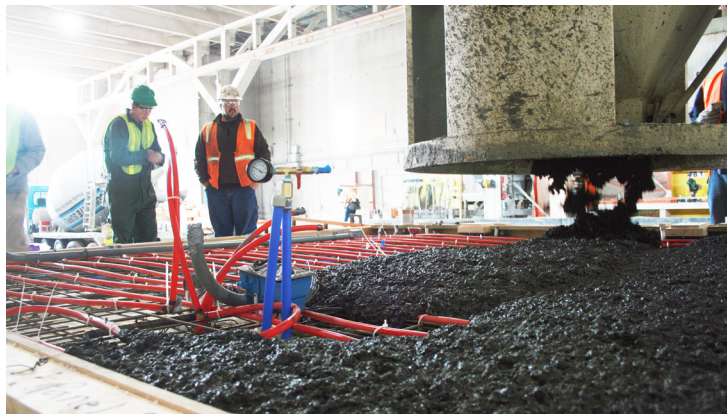
GCC precast wall panels were poured at a local plant showing that this technology is feasible now.
