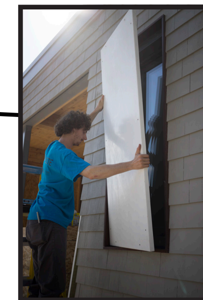
The same composite-panel technology used for the shutters was re-engineered to create strong, lightweight window plugs. A thin profile allows for easy storage, and simple hardware enables quick installation in response to a coming storm.
