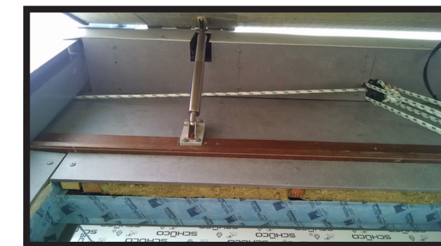
...most was off-the-shelf marine industry parts: pulleys, ropes, cleats, compression latches and gas springs.
