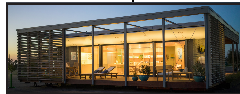
Shutters act as solar shades when open, and flood-proofing when closed.
